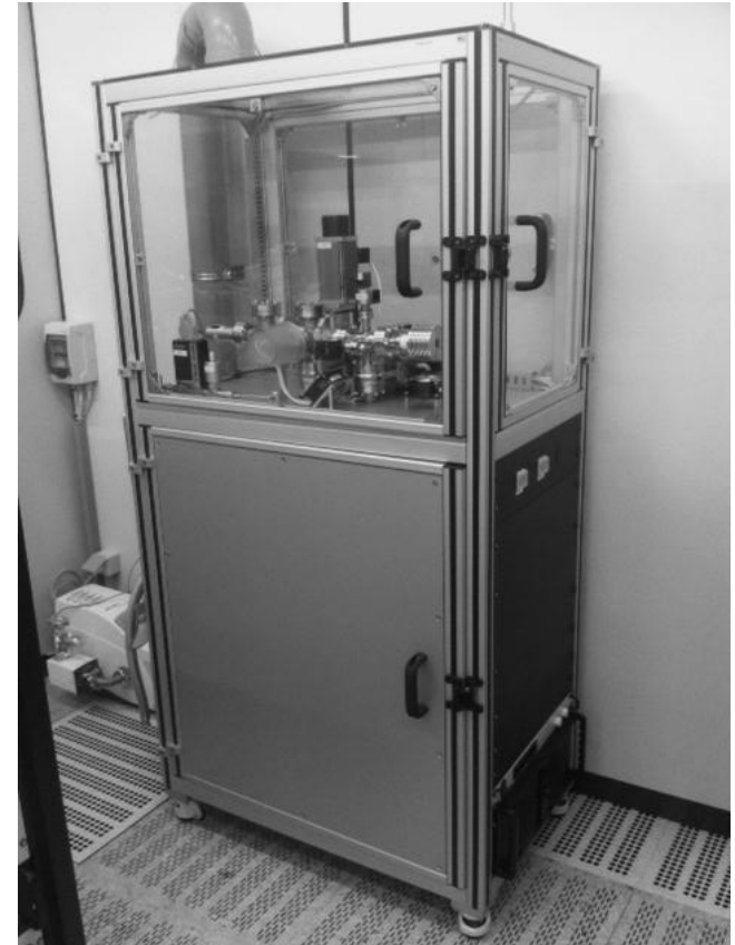
Installed at Imec Feb 8, 2012
